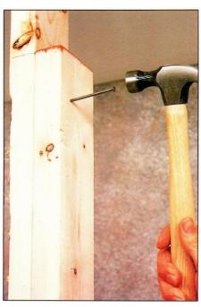
3 Nail the jack studs to the frame studs with 8d nails placed one foot apart from top to bottom.
