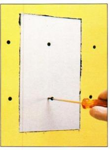
3 Place the new piece of drywall in the hole and fasten it to backer boards with screws. Press compound or fast-drying patching plaster into joints with joint knife. Tape joints (overleaf), and finish as shown below.
