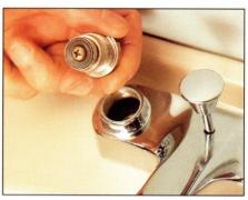
5 Inspect the rubber washer for wear. A worn washer will be grooved, pitted, frayed or cracked.
