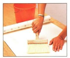
6 Brush paste onto the first strip starting at the top. If there is no arrow to indicate which end is up, turn strip over to check pattern.
