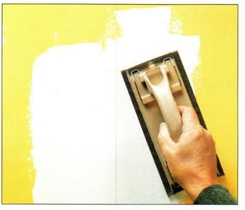
2 When compound is dry (at least 24 hours), sand with fine-grade drywall sandpaper on a sanding block. Wear a dust mask when sanding. If necessary, repeat these two steps until satisfied with your final surface.
