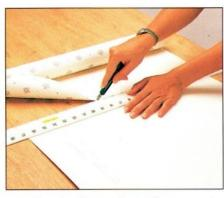
5 Cut the first strip to the correct length. Increase the length of subsequent strips as necessary to match patterns.
