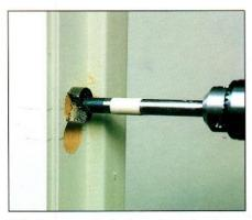
7 Bore two %-inch holes, % inch above and below the center line with a forstner bit (or spade bit), 1% inch deep into door jamb.
