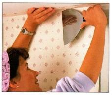
**5** Press blade of broad knife into ceiling joint to crease paper. Cut off excess paper along crease with utility knife, using broad knife as a straight edge. Wipe off excess paste.
