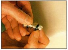
2 Replace the ring by rolling it on one end of the stem. The new ring must be the same size as the old to form an effective seal.
