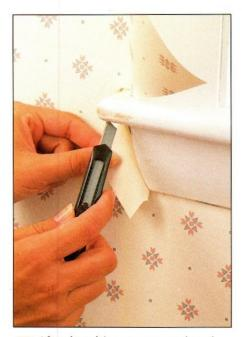
After brushing any completed sections into place, make whatever additional cuts are necessary to get an exact fit. Here, a horizontal slit is being made between the two sections of sill, one of which sticks out further than the other.
