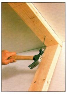
4 If the wall is parallel to and directly under a ceiling joist, nail the top plate to it. If perpendicular, locate ceiling joists and nail top plate to joists where they intersect every 16 inches on center.
