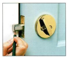
6 Trace bolt onto door jamb. Use a square and level to continue line around to inside edge of door jamb. Measure and mark the vertical center point where bolt will go into jamb.
