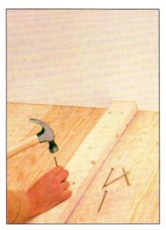
**3** Double nail (2 nails driven side by side) the bottom plate to the floor along the chalk line; use 16d nails. Begin a few inches from the wall and drive nails about every 16 inches along the plate through the subfloor.
