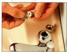
Turn the screw counterclockwise to remove the old washer. Clean the washer seat and stem by rubbing lightly with steel wool.
