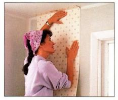
2 Allowing 2 inches to extend onto the ceiling, unfurl the top section, holding the right edge against vertical guide line. Press into place.
