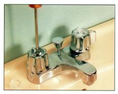
2 Remove the screw on the top of the handle and pull or pry the handle off. A decorative cap covers the screw on some faucets. Pry it off with a small screwdriver.
