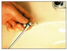
Pinch the O-ring and slide a knife or screwdriver blade beneath into the ring and pull it off.
