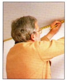
1 Measure along edge of ceiling from the top of existing wall to the point where one end of new wall will intersect, and mark with a pencil. Repeat this step at the opposite end of the room.
