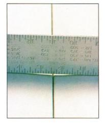
The two long sides of drywall are tapered to create a trough when placed edge to edge, so that joint tape and joint compound can be applied without bulging out too far beyond the wall surface.
