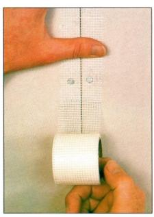
4 After nailing or screwing in place along the top and bottom plates and studs every 16 inches, apply fiberglass joint tape to the seams, with the sticky side to wall.
