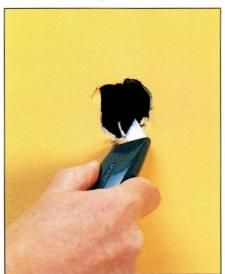
1 Clean away loose drywall and cut off loose paper. Leave the inner surface of the gypsum rough. Cut screen 2 inches larger than hole all around. Tie one end of 12-inch string to a small stick; thread other end through center of screen.
