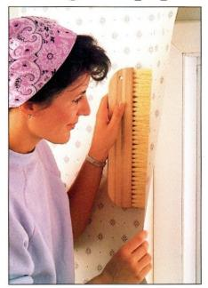
1 Wallpapering around door and window frames is tricky. Precutting to fit is the riskiest way to deal with these obstacles. Instead, put up a whole strip of wallpaper and brush it into place as far as the point where the wall meets the obstacle.
