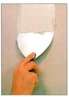
5 Apply joint compound over tape with 6-inch broad knife and smooth out over the seam by holding handle at a tight angle to the wall. Let dry at least 24 hours, sand, and repeat process using 10-inch broad knife. Let dry and sand.
