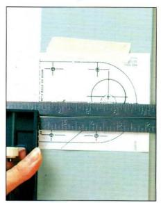
Tape the template that came with your lock to the inside edge of door, following guide lines. Use straightedge and level to ensure it is placed correctly and perfectly level on the door.
