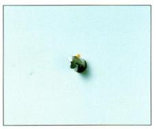
4 Drill only deep enough for the guide bit to poke through the other side of the door. Then finish drilling from the outside. This prevents splintering the wood.
