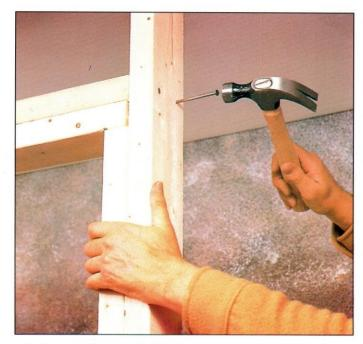
4 Cut two 2x4s each 35½ inches long (for a 30-inch door) and nail them together. Place this double header on top of the jack studs. Secure them by driving two 16d nails through each side of the door frame studs.
