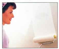
1 Apply oil-based primer which dries to a hard finish, to protect walls from moisture and make stripping easier later. Let dry and sand lightly.
