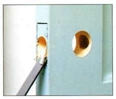
3 To recess the bolt plate flush with the door edge, shave away the wood in thin layers with a chisel. For a sharp outline to the mortise insert the bolt assembly and score around the plate with a utility knife.
