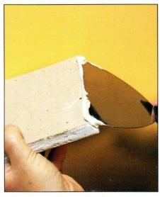
2 After adjusting fit, if necessary, with a utility knife, spread compound along the beveled edges of the patch. Fit patch in place with light pressure. Matching bevels prevents patch from falling through.
