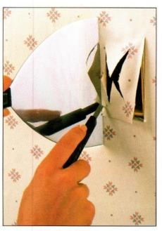
10 While holding the broad knife against the outlet to form a straight edge, trim the paper around inside edges with utility knife. Replace the faceplate.
