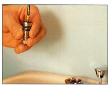
2 Replace the old washer with a new washer of exactly the same size. Do not overtighten the screw as it will compress and deform the washer.
