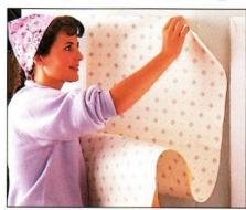
1 Drape pasted paper over your arm as shown and carry it to the wall. Install the top of paper just over the ceiling line.
