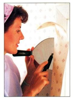
4 Trim the vertical edge next, using broad knife and sharp utility knife. Follow the corner formed where the wall meets the frame.
