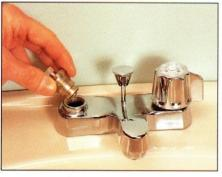
4 Unscrew the stem by turning it counterclockwise. Lift it out of the faucet body.
