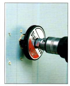
Insert the 14-inch hole saw or, as here, an adjustable hole saw in your drill. Position the center guide in the hole you punched for the cylinder. Hold drill very straight and begin drilling. Use a drill guide or have an assistant help you.
