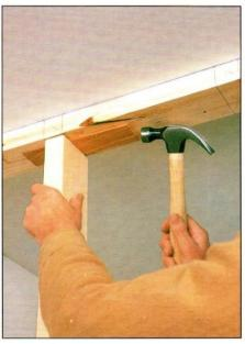
5 Measure and cut studs individually. Nail them into top and bottom plates where marked. If a stud is cut a little short, shim it at the top plate with a piece of wood shingle.
