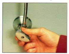
Turn off the water supply by turning the shutoff valves clockwise. Shutoff valves are usually located under the sink, but may be in the basement instead.
