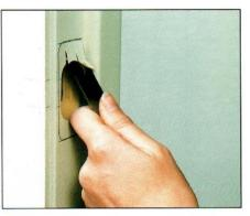
9 Align strike plate on the jamb and scribe around it. Mortise about ¼ inch deep, until strike box and its reinforcing plate fit snugly.
