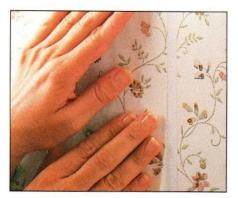
Position subsequent strips on the wall about ¼ inch away, then slide them gently into place. If the paper does not slide very easily, gently lift and reposition, then brush.
