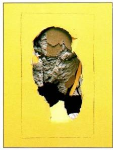
1 Measure hole. Cut a rectangular or triangular patch from a piece of drywall making it at least 1 inch larger than the hole on all sides. Trace patch onto wall and cut out shape using saw or utility knife.
