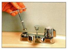
1 Insert the valve seat dressing tool into the housing of the faucet and lower the retaining nut so that it holds the tool straight.
