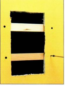
2 Insert a backer board with construction adhesive applied to the ends. Holding firmly in place, screw drywall screws through drywall into board, at least 1 inch away from edge of hole. Repeat if using two backer boards.
