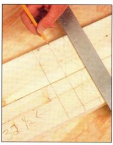
2 Mark the location for the door. The rough opening (r.o.) for any door is 2½ inches wider and 1¾ inches higher than the door itself. Door sizes vary, but a common size is 30 inches by 6 feet 8 inches. Using a 30-inch door, the r.o. would be 32½ inches by 6 feet 9¾ inches.
