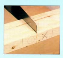
☐ When you mark the rough opening on the sole plate, you will have 3 lines showing placement of the wall stud and placement of the jack stud butting it. At the middle line, cut halfway through from the bottom side of the plate. When you remove this section of the sole plate from the doorway later, you can cut through from the top without marring the floor.
