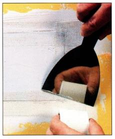
3 Smooth the compound and apply drywall tape over all joints with the joint knife. At end of each joint, press edge of knife blade in firmly and use as straightedge to tear off tape. Sand when dry.
