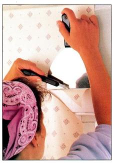
3 Brush horizontal section into place. Crease into corner with back edge of broad knife and trim with sharp utility knife against the blade of the broad knife still pressed into crease.
