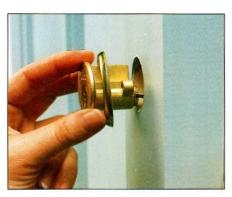
5 Place the cylinder ring around cylinder. Then insert the cylinder and connecting bar into hole from outside of door. Position keyhole at bottom, trademark at top. Hold cylinder in place.
