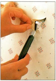
Always turn off electricity when working around switches and outlets. Remove plates. With current still off, hang paper. Make X-shaped slits over exposed fixtures.
