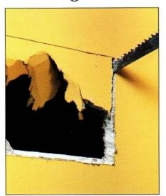
1 Measure a rectangular drywall patch about an inch larger than the hole. Cut it at a bevel with drywall saw, or use a saber saw with angled base plate. Use patch as a template to mark wall, and cut around hole at same bevel as patch.
