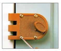
7 Set bolt in unlocked position. Fit the connecting bar into its slot on back of bolt. Attach bolt to inside of the door using the screws provided. Check that bolt works from both sides of door.
