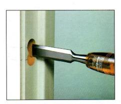
8 With a chisel, work the wood out between the two holes to form one long hole in which the strike box will fit.
