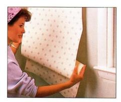
4 Fold out the bottom half; hold it in place along vertical guide. Press and brush quickly. As paste dries, it is harder to remove bubbles.
