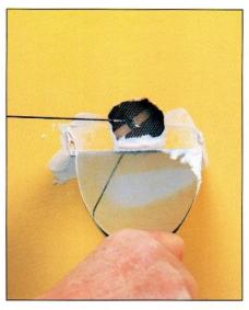
2 Bend screen and insert stick and screen into hole. Pull on string so the stick holds screen flat against back of hole. Holding string taut, fill hole, working in from the edges. Make sure compound adheres to mesh. Tape string tightly against wall with masking tape.
