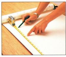
4 Measure the height from the baseboard to the ceiling. Mark off this distance plus 4 or 5 inches on the first strip of wallpaper.
