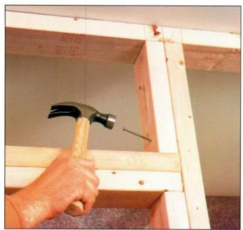
**5** Measure the opening between the top of the header and the top plate, and cut three cripple studs. Nail one against each frame stud, and center the third over the door opening.
