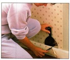
6 Brush strip again and trim excess paper at bottom with sharp utility knife, using broad knife as straight edge.
