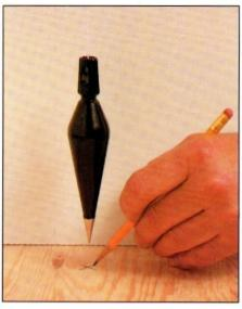
3 Drop a plumb bob from each end of chalk line to floor and mark with an X. Snap a line between the two points to mark edge of sole plate. Snap lines on walls connecting ceiling and floor lines.
