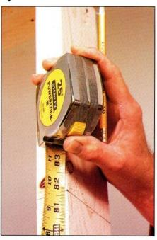
2 Measure and cut the two jack studs to be 1¾ inches longer than the height of the door.
