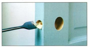
After following Steps 1 to 4 for installing a surfacemounted deadbolt to mark and drill cylinder hole, drill bolt hole through side of door. Use %-inch drill bit or appropriate bit for your particular lock; be sure to drill straight.
