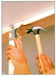
6 Fasten each stud to the plates at the top and bottom with metal connectors, using 8d nails. Alternately, toenail the studs to the plates (right), using 16d nails. While working, use level to check that studs are plumb.
