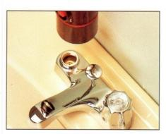
6 Inspect the valve seat by looking down into the faucet body with a flashlight. If the seat is scored or pitted it will need to be reground or replaced.
