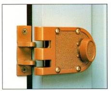
Once the lock strike is in line with the lock, check to see if the lock strike needs to be shimmed or mortised into the door jamb, or if it sits correctly on the surface. Mortise if necessary and screw into place.
