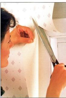
2 At the top or bottom of the door or window frame, cut the wallpaper with scissors diagonally (miter-cut) to permit separation into two sections: one to extend along the side of the frame, the other horizontally.
