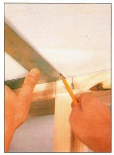
1 Lightly mark the center of each stud location on the floor and ceiling with pencil. This will provide you with the lines for nails or screws when drywall is in place.
