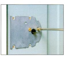
6 Position backplate on inside; insert screws through plate into screw holes in cylinder. Plate will sit ¼ inch from door edge. Connecting bar will extend through hole; break it off as described below.
