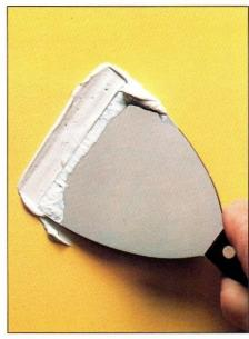
Joint compound for dents. Clean off loose edges. Dip joint knife into compound sideways and load about half the blade width. Pull knife across dented area with a slow smooth stroke. Position knife at a 90-degree angle to the first stroke and pull across again to remove excess compound. When dry, sand to finish.
