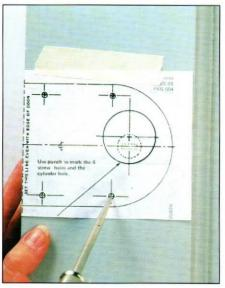
Shut door or wedge firmly. With awl, punch holes for drilling where template indicates for the four screw holes and center of cylinder hole. Use the 1/8-inch drill bit and hold drill straight to drill the 4 screw holes, 34 inch deep.
