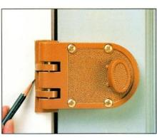
8 Set lock strike in bolt in locked position. Mark the vertical measurement on door jamb. Then move the lock strike up so the latch bolts are centered and mark the top and bottom measurements.
