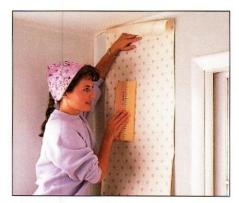
3 Brush to make the paper stick to the wall and drive out air bubbles. Work from the top down and from the center to the sides.
