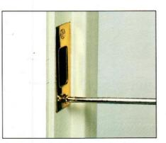
10 Install strike box and reinforcing plate. Mark holes for the screws and drill with 3/16-inch bit. Use 3-inch screws, so strike cannot be torn from the door with a sharp kick.
