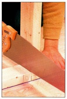
1 Saw through the top of the sole plate at the inside edges of the king studs, to meet the cut you made earlier in the bottom. Remove the cut portion of the plate.
