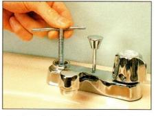
2 Turn the handle clockwise a few times while applying light downward pressure. Work slowly and carefully. Your goal is to smooth the seat, not to grind it down.
