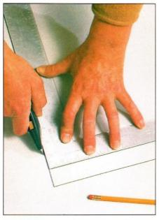
2 After measuring and marking, cut the drywall with the utility knife along the face of the sheet, using the framing square as a guide.
