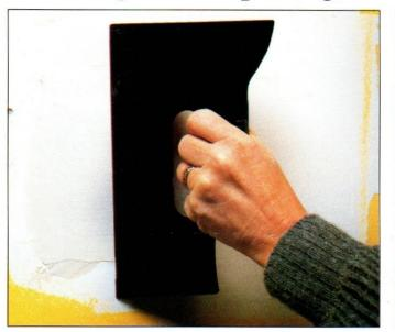
1 No matter how small or large the repair, the method for finishing is the same. With wide joint knife spread a smooth, thin layer of joint compound over the repaired area or over all joints of new patch. Extend beyond edges of repaired area and feather out to surrounding wall.
