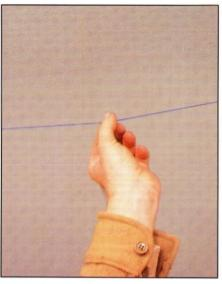
2 Drive a nail halfway at the mark at each end. Stretch a chalk line between the nails and snap it. This marks the line for the outside edge of the top plate on the new wall.
