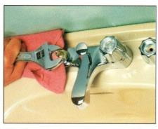
3 Remove the packing nut with an adjustable wrench, turning counterclockwise. Use a rag, masking tape or other padding material to protect the fixture.
