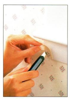
**8** Make final paper cuts only after you have been able to brush the paper into place against the obstacle. The loose vertical section alongside the window frame can now be easily trimmed.
