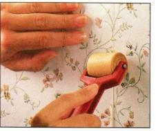
8 After the paper has been up for 10 to 15 minutes, press seams firmly with a roller. Wipe off excess paste with a towel.
