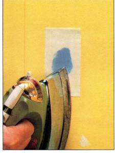
Iron-on patches for small holes. These patches are a new method for repairing small flaws in drywall. Cut the polymer fabric to size and iron with a household iron set at medium heat. Apply compound over fabric and sand when the compound has dried. Always wear a dust mask while sanding joint compound.
