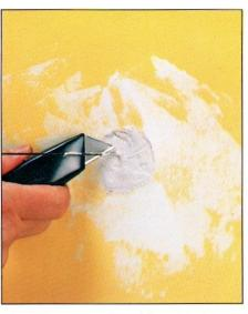
When compound has dried completely, cut string flush to wall. If using joint compound, remember it will shrink; apply another layer to bring patch up to surface of wall. You may have to apply a third layer. Then proceed to finishing as shown (overleaf).
