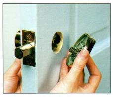
5 Rotate connecting bar to vertical position and install thumbturn. Secure with mounting screws. Make sure bolt projects and retracts easily.
