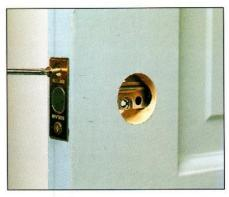
4 Install latch bolt plate and screw into place. Insert cylinder into hole on outside of door, sliding connecting bar through its slot. Bar will extend to inside of door.
