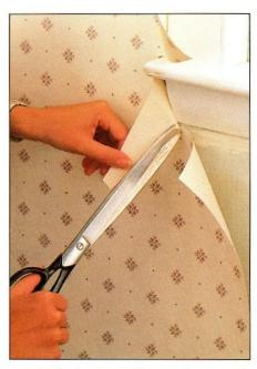
6 Make horizontal cuts above and below the obstacle, to the end but not beyond the obstacle. Use scissors for the larger initial horizontal cuts to the edge of the obstacle. Use a utility knife to make the smaller horizontal cuts.
