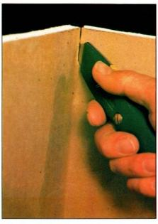
3 Break the drywall along cutline with a gentle snapping motion. Fold it up and cut the paper along the back of the sheet.
