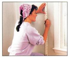
3 To start papering, use the level to establish a true vertical guideline from floor to ceiling one width of the roll plus 8 inches away from an inconspicuous corner.
