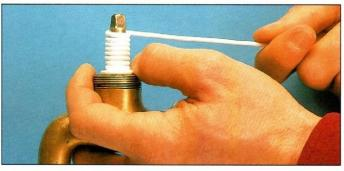
**Packing string.** Remove old packing string from the stem and wrap a few turns of new packing string around the stem. Replace packing nut on stem and tighten; this compresses the packing to prevent leaks. Do not overtighten.
