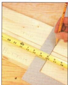
Measure the ceiling and floor lines and cut the top and sole plates. They may not be exactly the same length, so label the boards as "top" and "bottom." Mark the placement for studs every 16 inches using a framing square.
